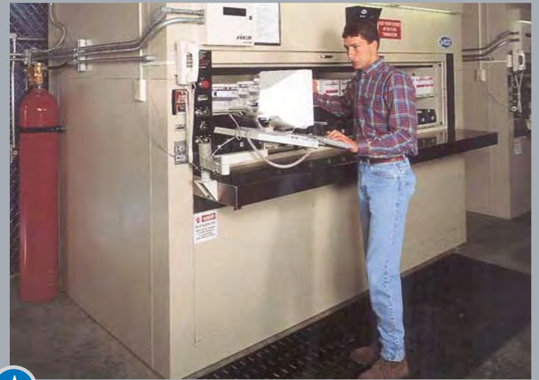
Environmentally friendly CO 2 fire suppression system protects vertical carousel system
